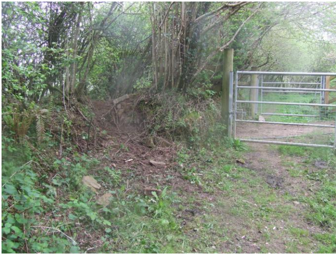
13 Bank damage at Wooda Bridge
