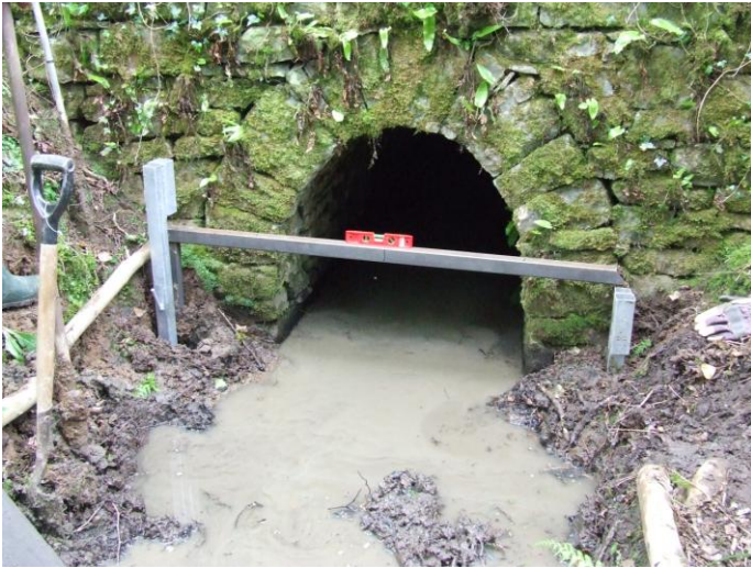
16 Gate retaining posts
