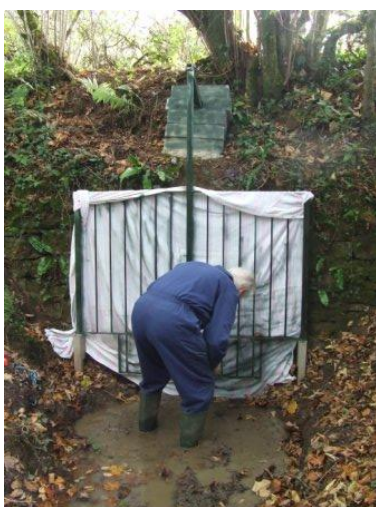
12 Entrance protection whilst painting gate
