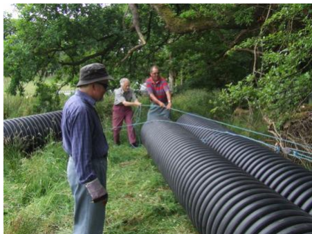
1 On far side of stream
