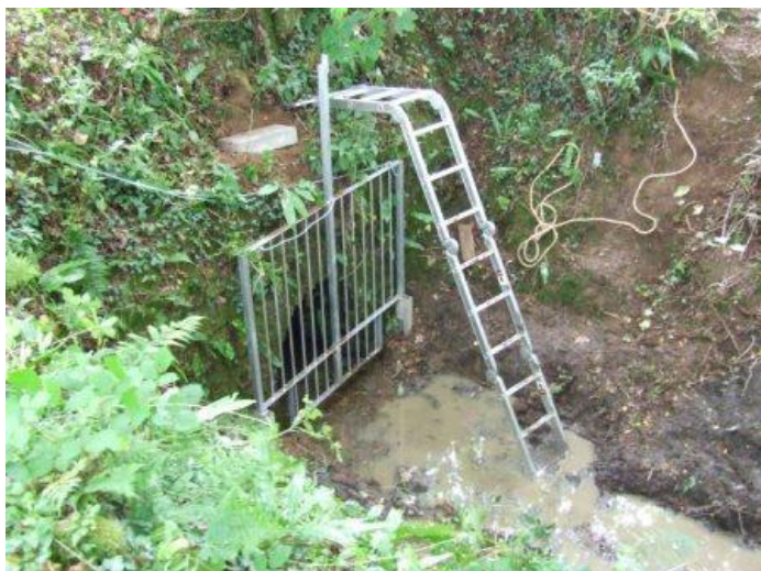
9 Securing the adit gate
