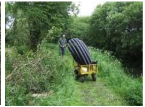
12 culvert liner pipe
