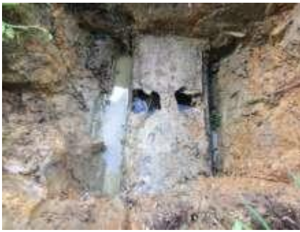
7 slots cut in clay to take support
