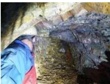
13 loose stones and solid wall
