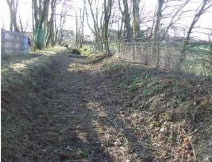
10 – Aqueduct bridge cleared of vegetation
