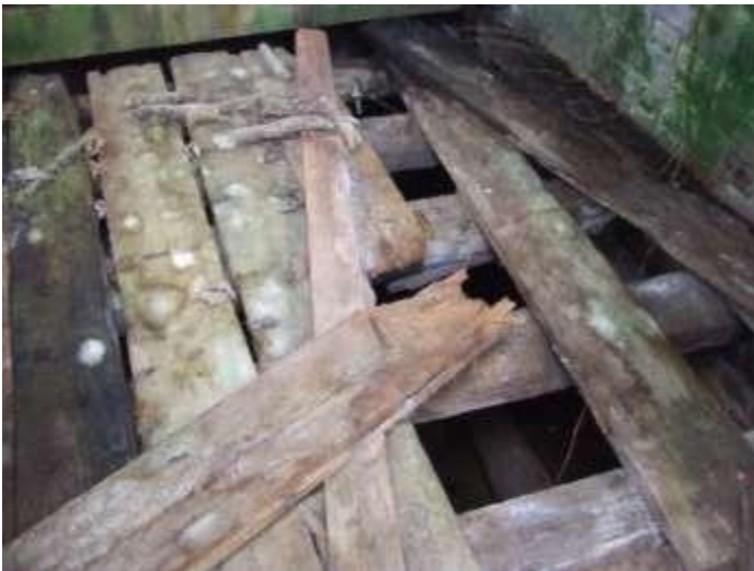
12 – View inside door
