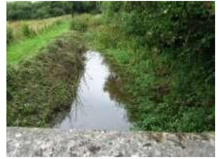
9 north side started
