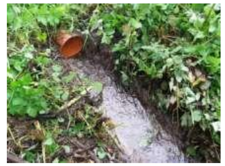
6 pipe to next section cleared
