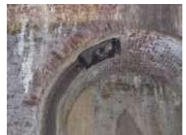
4 Roof and exit in chainwheel chamber
