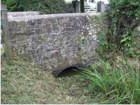
22.Strimmed south side of Vealand Bridge
