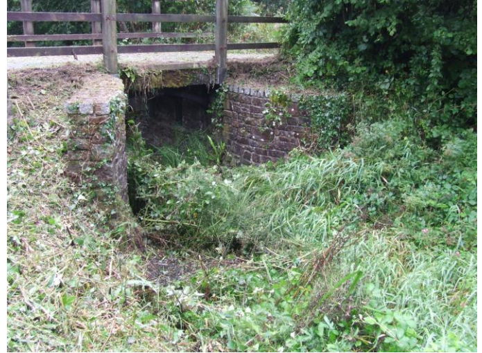
16.Moreton Bridge semi-cleared
