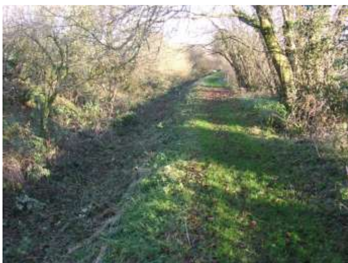
12.Looking back at completed clearance
