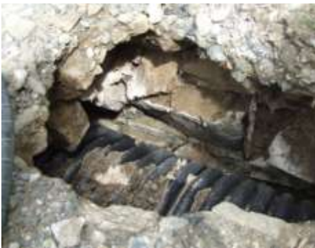
9. Collapsed culvert
