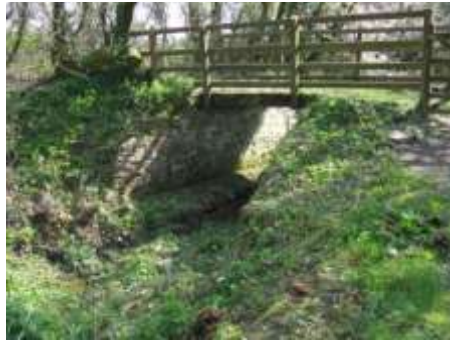
2. Broomhill North side cut
