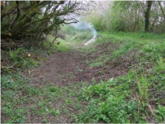
7. Clearing and burning at Aldercott
