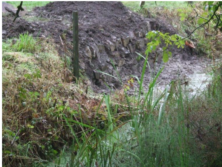
25.End of the first day's work
