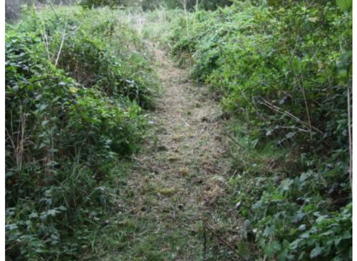
17 Attempted cut into Filter bed overgrowth
