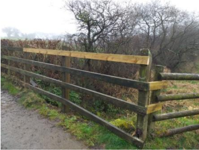
26 Replaced rail and post support at Lana
