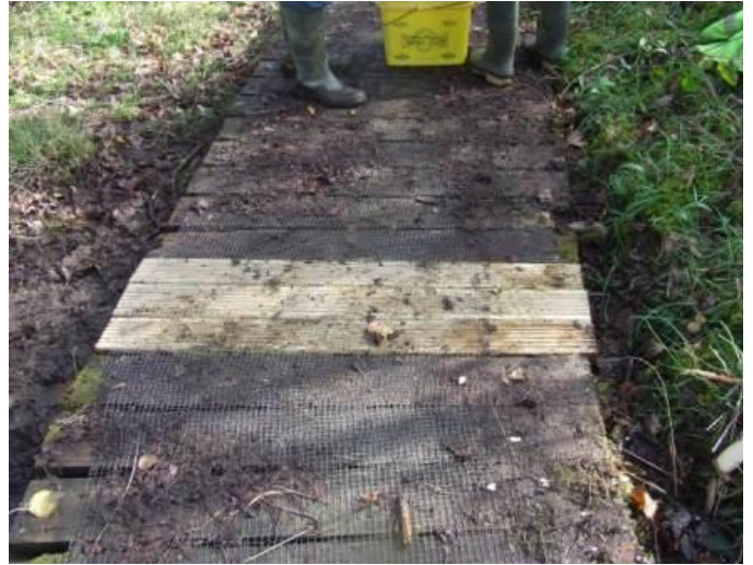
27 Old boardwalk plank repairs
